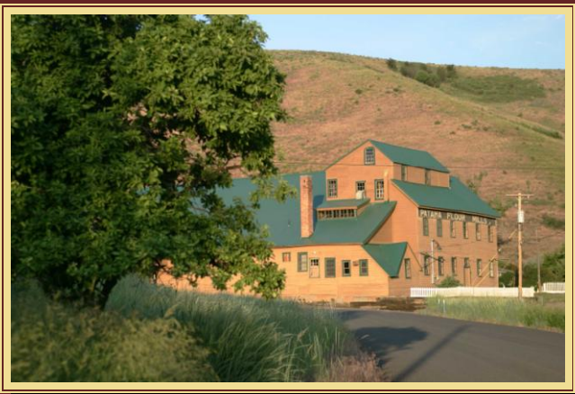
HISTORIC FLOUR MILL, GARFIELD COUNTY
